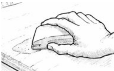
Figure 23 Sand cured fairing compound to desired contour.
